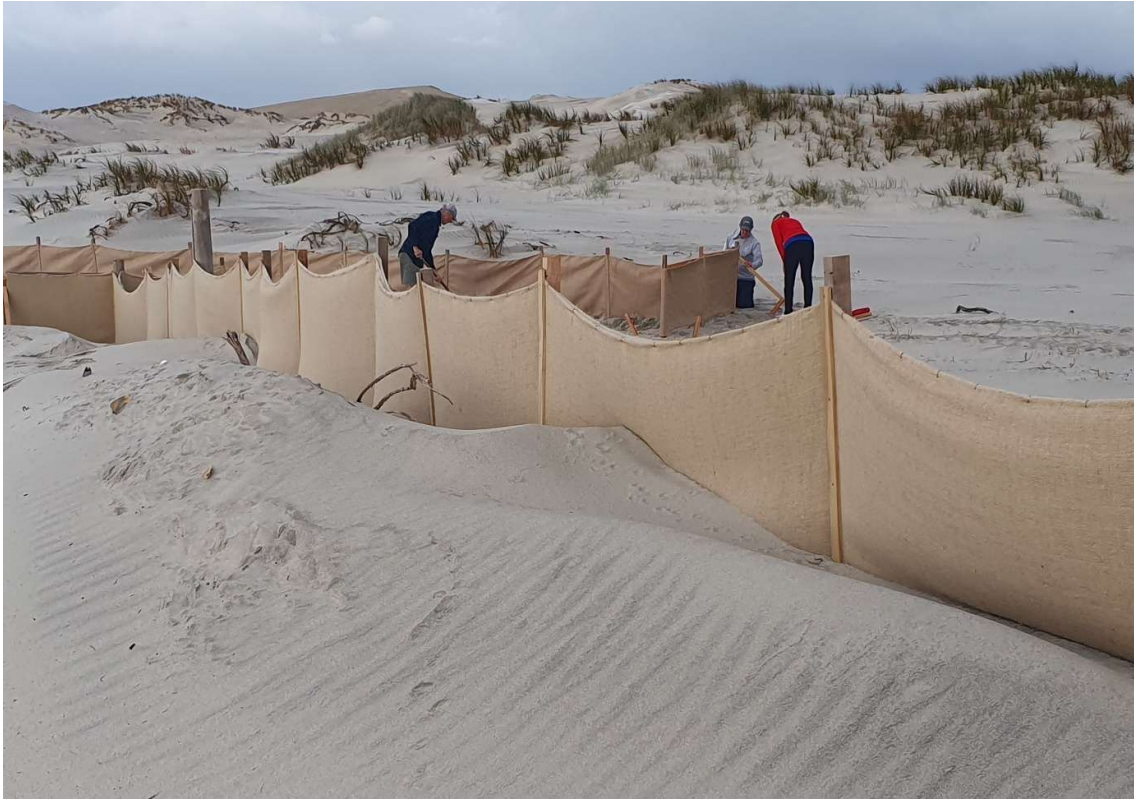
Sand fences being erected – 2025.
