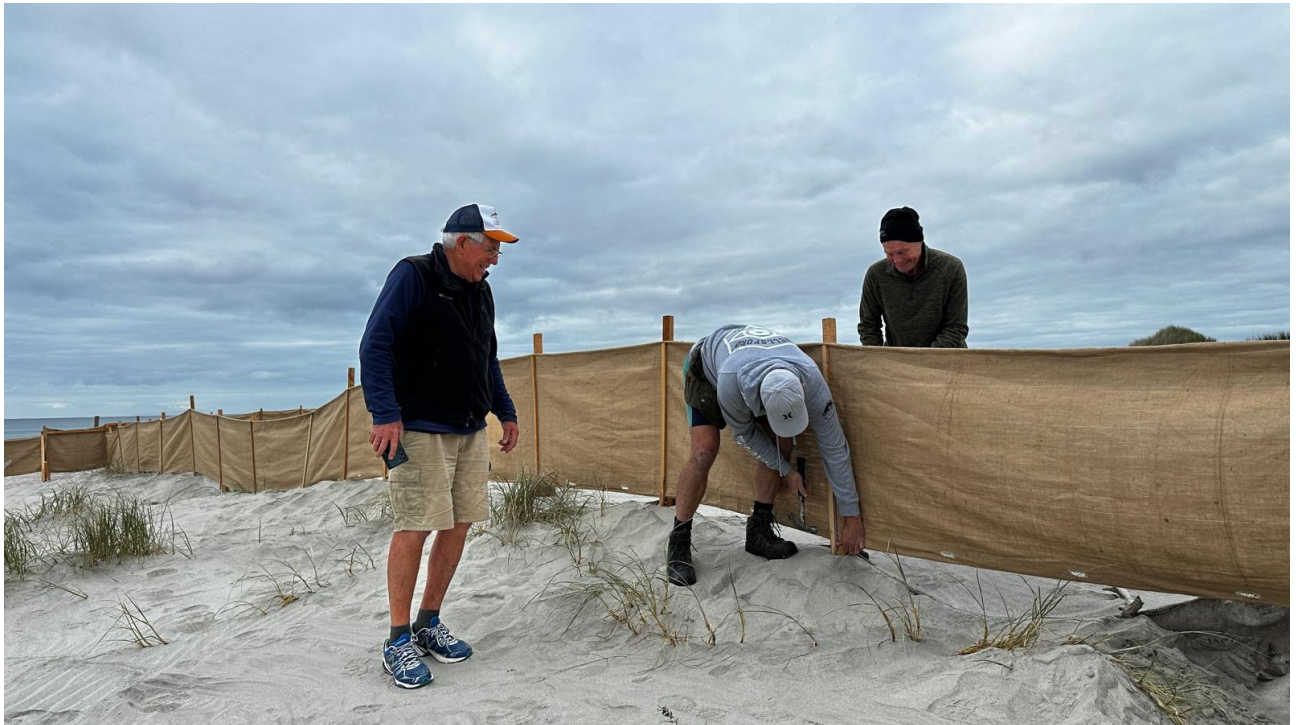
Part of the 275m of fence that was restored
