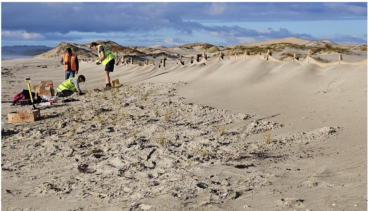
Planting taking place along the fenceline – note sand buildup on fence after only 3 weeks.
